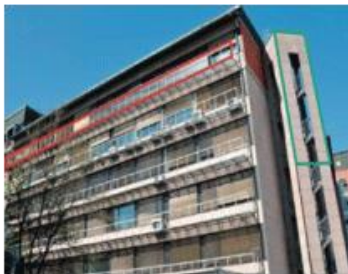
Fig 11: Office Building in Ljubljana, Slovenia (Zhang X et al. 2015)
