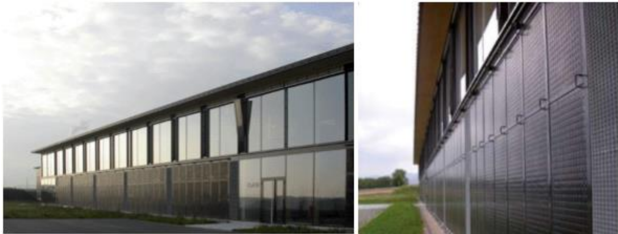
Fig 6: Solar integrated on the Centre d'entretien des Routes Nationales (CeRN) in Switzerland (Rafaella Agathokleous, 2014).
